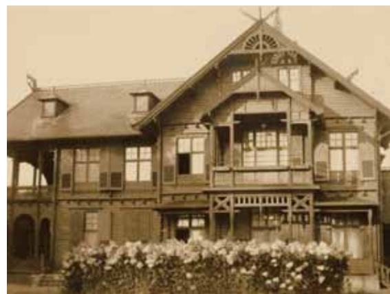
Timber-framed estate house Kemperberg
