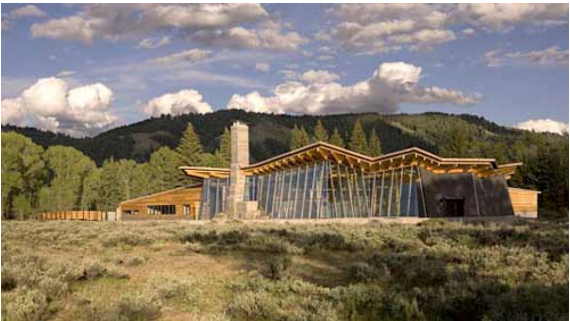
The Capitol Reef National Park Visitor Center (above) and Grand Teton National Park Visitor Center (below) are American examples of distinct yet respectful architecture based on the landscape
